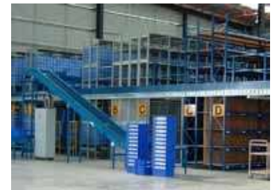
MK 197 Mezzanine Floor Racking System
